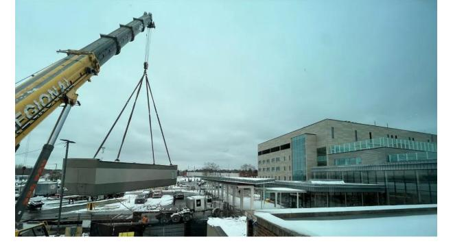
After 10 days, more than 1,700 kilometers, and the transportation of two 130-foot tractor-trailers, the two specially designed building units for the new Brockville General Hospital MRI arrived on March 23rd. Each unit, weighing approximately 110,000 pounds, was carefully lifted into place by crane throughout the day. With both units now on-site, the next phase of connecting electricity and plumbing to the hospital has begun.
